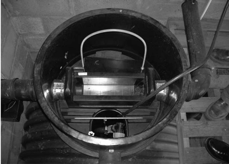
Plate 3.2. Manhole access showing filter (Photo: L. Fewtrell)
